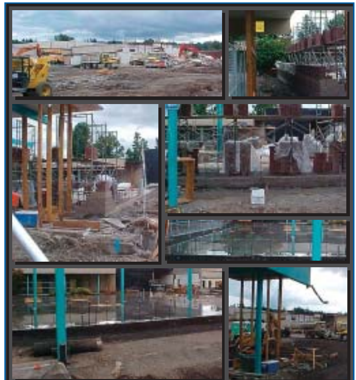
Sweet Home Center Remodel Under Way
